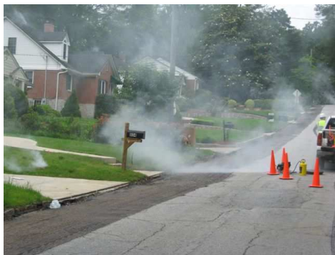
Typical smoke testing blower and smoking defect.
