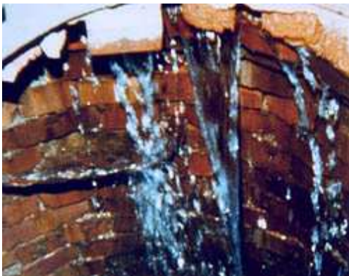
Inflow entering the sewer system through a manhole.
