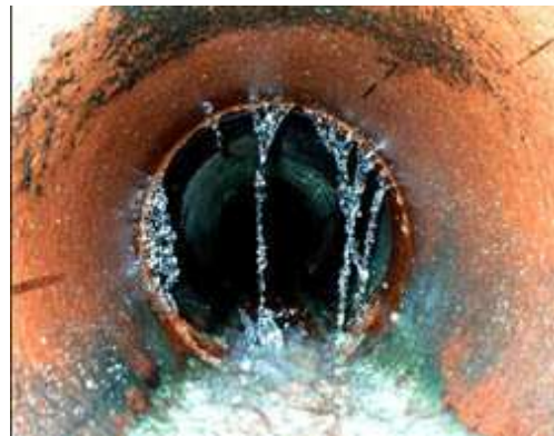
Infiltration entering the sewer system from a pipe defect.
