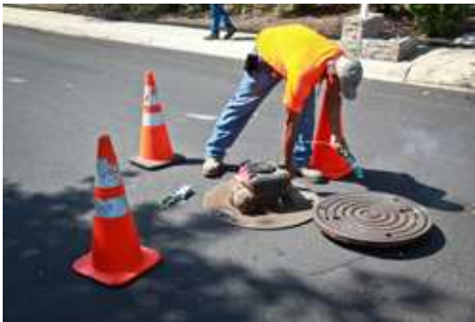
High-capacity blowers are used to pump smoke into a manhole.
