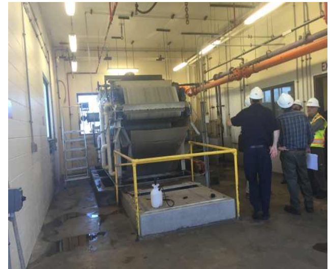
SLUDGE BELT THICKENER/PRESS
