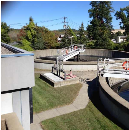
FINAL SETTLING TANKS
