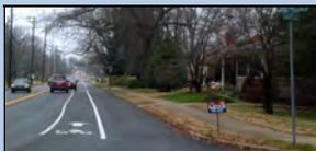
**Narrowing Travel Lanes** - Narrowing travel lane width can calm traffic. A constriction (choker, chicane, etc.) can also be effective although it can hamper snow-plows and emergency response.
