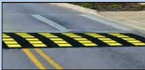
**Speed Bump / Hump** – Temporary or permanent raised sections of roadway which can deter speeding and cut-through traffic. However, this can also create issues for snow plowing and emergency response.
