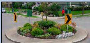
**Mini-Roundabouts** - A mini-roundabout is a street intersection feature which requires vehicles to slow down and navigate around the island in an intersection and yield to vehicles already in the roundabout.
