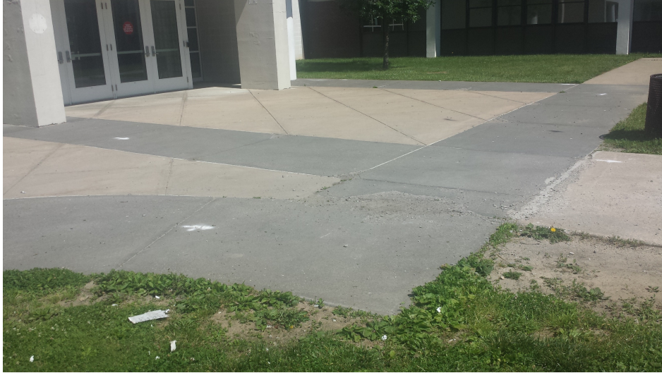
Tinted Concrete Sidewalk Replacement Adjacent to the Building
