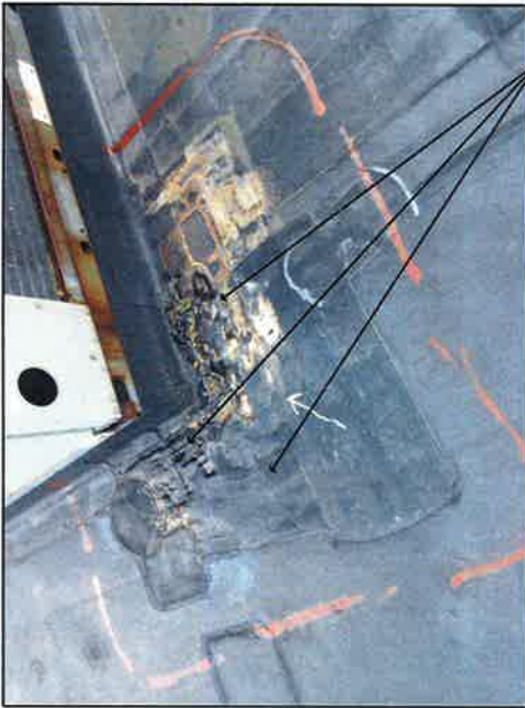
I CONTAMINATED EPDM AT ROOF 13 R2
