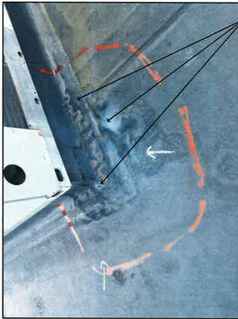
H CONTAMINATED EPDM AT ROOF 13 R2
