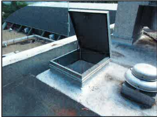
E R5 ROOF HATCH
